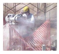
his employer who subsequently hired an outside firm to collect air samples of the work area. The samples contained about 200 times the NIOSH Recommended Exposure Limit (REL) for crystalline silica. The type of respirator the worker was wearing had an Assigned Protection Factor (APF) of 25, which provided protection from hazardous concentrations only up to 25 times the NIOSH REL. Estimate the causes of the accidents in this situation. Design a prevention system for this exposure.
